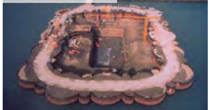
Bridge construction, South Korea
