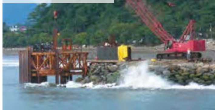
Marina breakwater, Costa Rica
