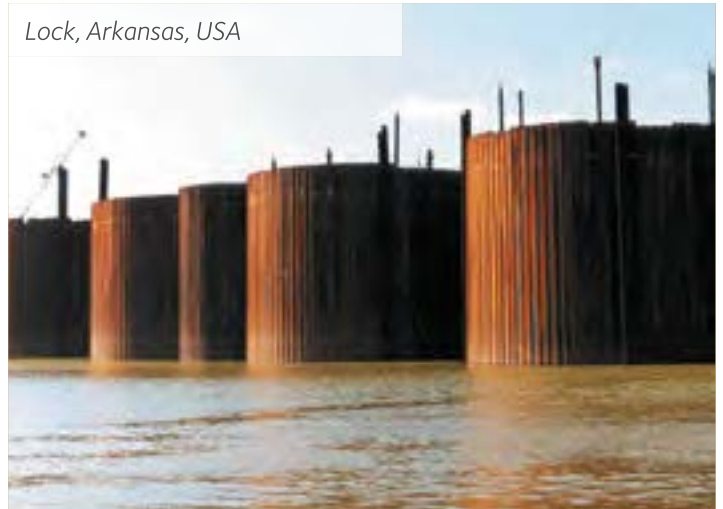
Diaphragm cells with 120^\circ junction piles.
