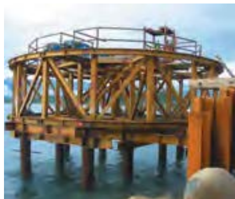
1. Installation of template
