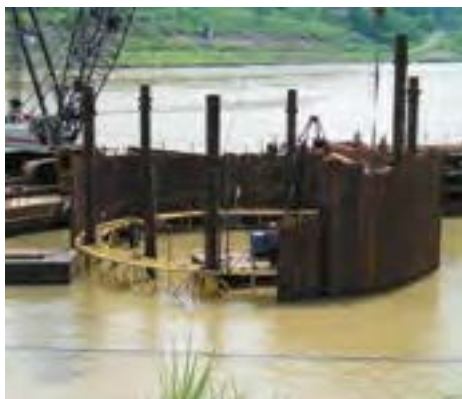
2. Threading until cell closure
