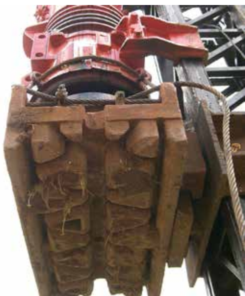
Position of section HZ 880M / 1080M / 1180M as box pile
